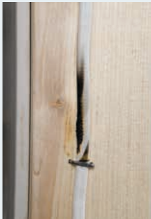
Damaged wiring
